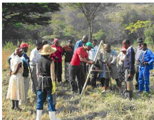
Plate 2.3a - Trainees setting out a swale at NMPLC
