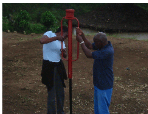
Plate 2.4f - Demonstrating the fence post hammer
